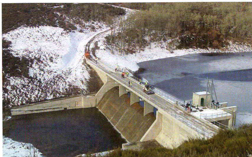
Views of the dam and fish pass at the Canedo hydro project in Portugal
